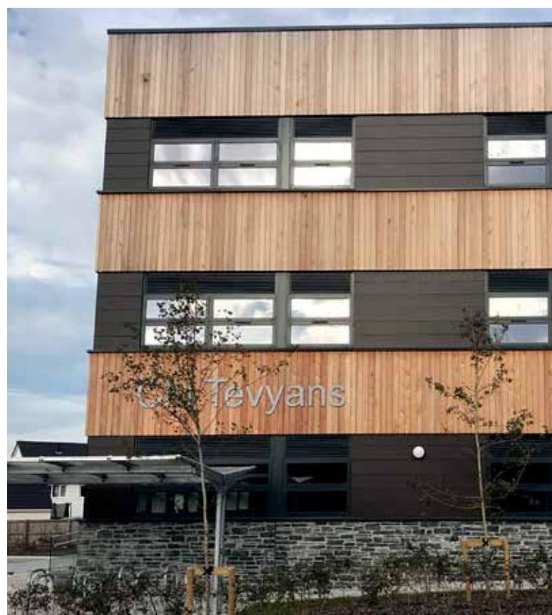
An example of the use of thermally modified wood in facades
