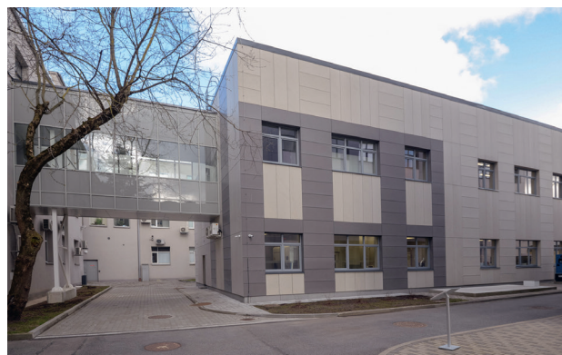
The building of the Biotechnology facility
